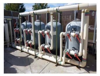
These are Astral pool filters with a filtration area of 12.16ft.2. Model #06683. According to the equipment sticker these filters were installed in 2009.
