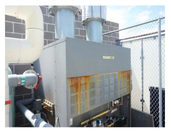
This is a Pentair Mega Therm natural gas commercial heater with 2,800,000 BTU/input located in the equipment area.
