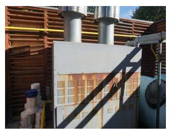
This is a LAARS natural gas commercial heater with 2,800,000 BTU/input located in the equipment area.
