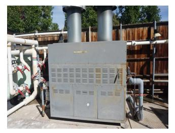
This is a Pentair Megatherm commercial heater with 3,200,000 BTU/input located in the equipment area.
