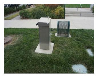
These are the backflow devices located throughout the community. This is for the replacement of three (3) backflow devices every year. This component, and all information contained herein, has been provided by the clients contractor and incorporated into this analysis at their request.
