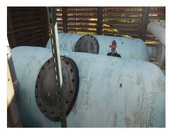
These are Astral pool filters Model #11330. According to the equipment sticker these filters were installed in 2003.
