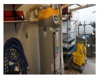
This is a A.O. Smith Cyclone xi 100G natural gas water heater located in the equipment area.
