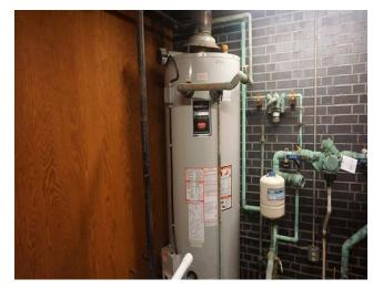
This is a State 100G natural gas water heater located in the equipment area.
