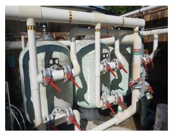
These are Astral pool filters with a filtration area of 12.16ft.2. Model #06680. According to the equipment sticker these filters were installed in 2007.
